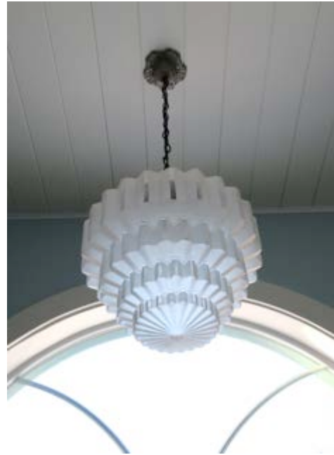
Three light fixtures like this one survived the fire. They've been rewired, cleaned up and are back in place.
