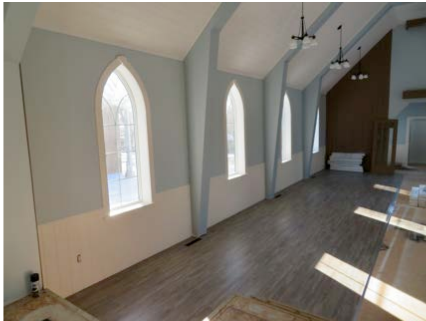
Great care was taken to have the replacement windows look as much like the old ones as possible.
