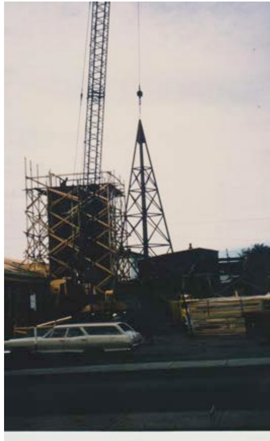
Bell Tower Takes Shape November 1965
