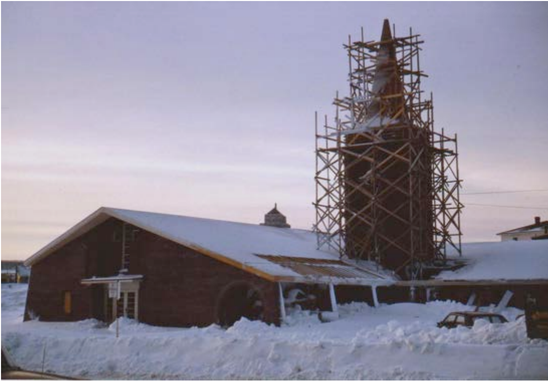
Bell Tower Attached
