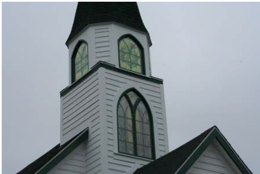
Windows in the New Steeple
