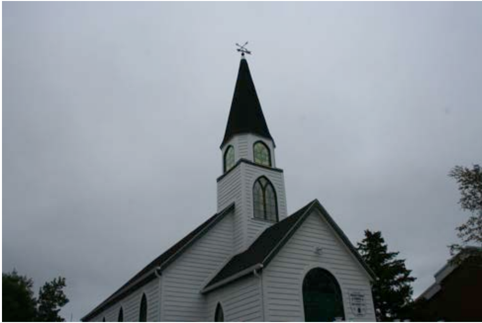
New Steeple with Weather-vane
