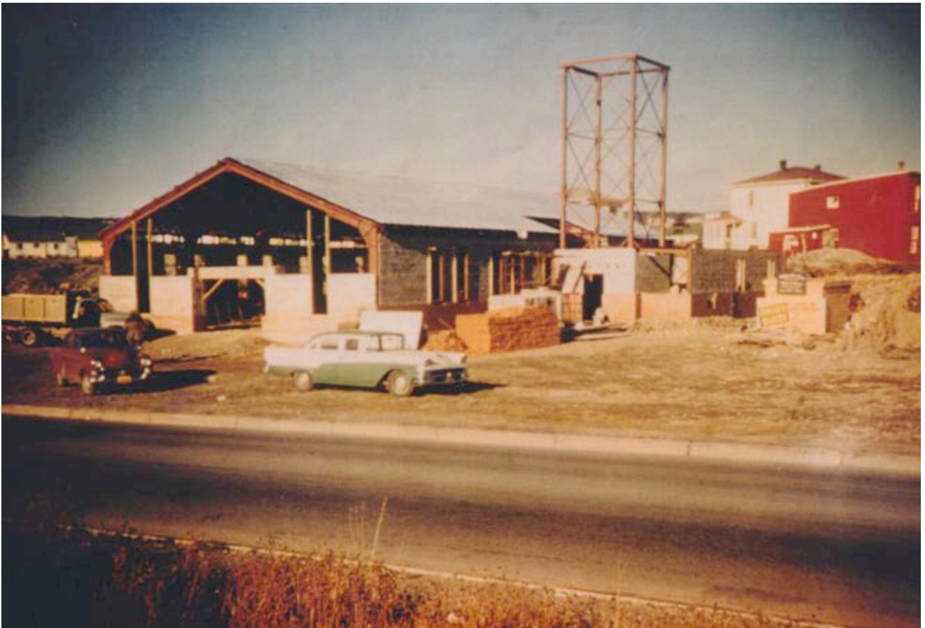
St. David's Under Construction – 1958
