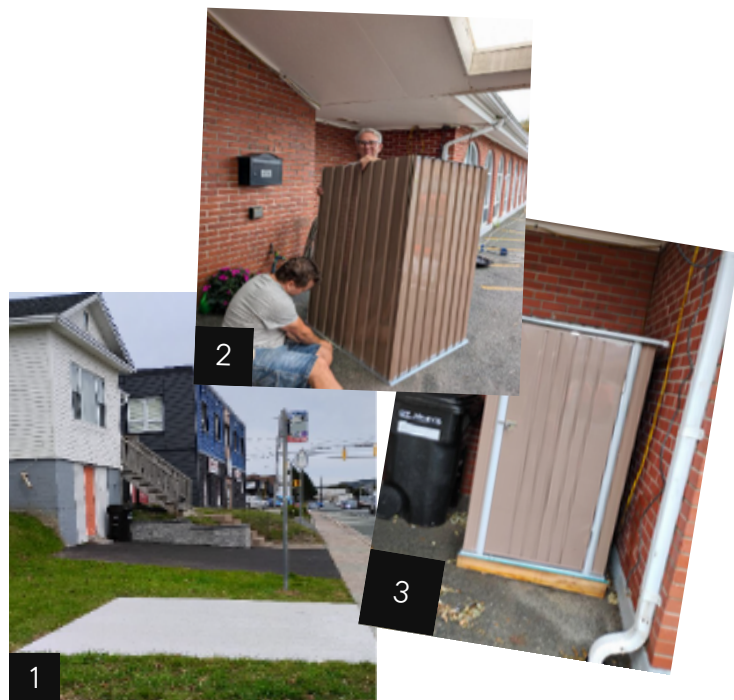
1: The new bus shelter progress 1: Building the shed 3: The final shed product!
